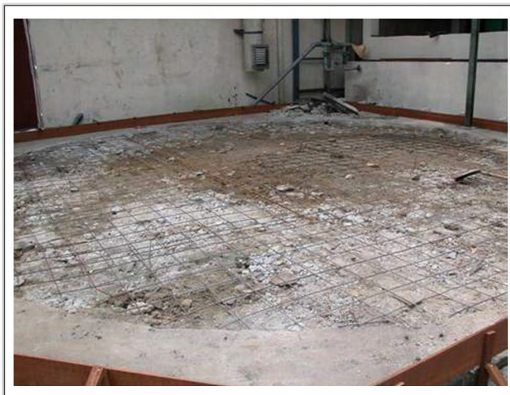
Additional A8 BRC Being Laid @ Center Sedimentation Tank
